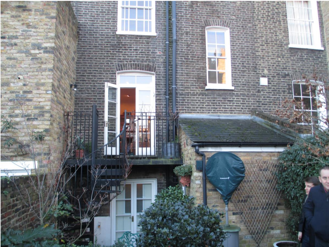
Image 5 – View of rear elevation at basement level
