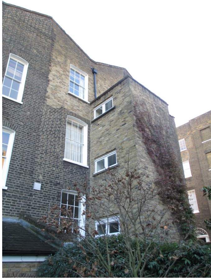
Image 7 - View towards rear elevation of no. 51 from rear garden
