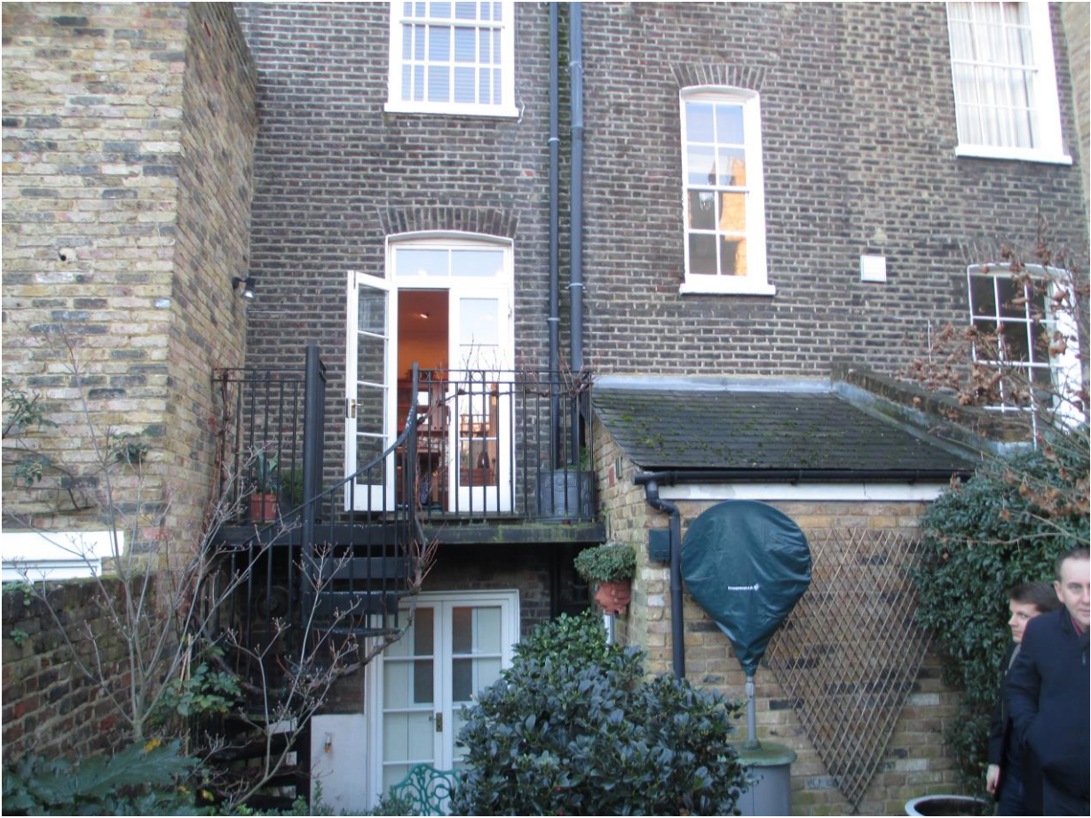
Image 5 - View of rear elevation at basement level
