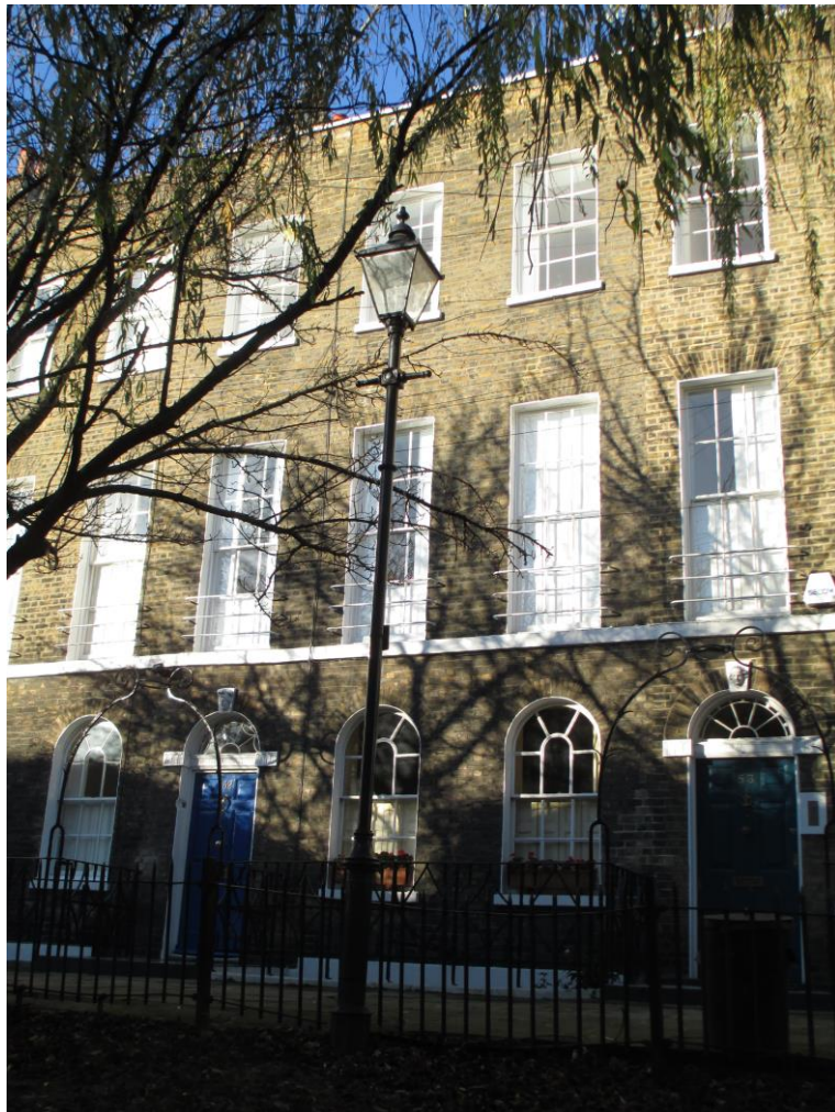
Image 2 - View of front elevation of site
