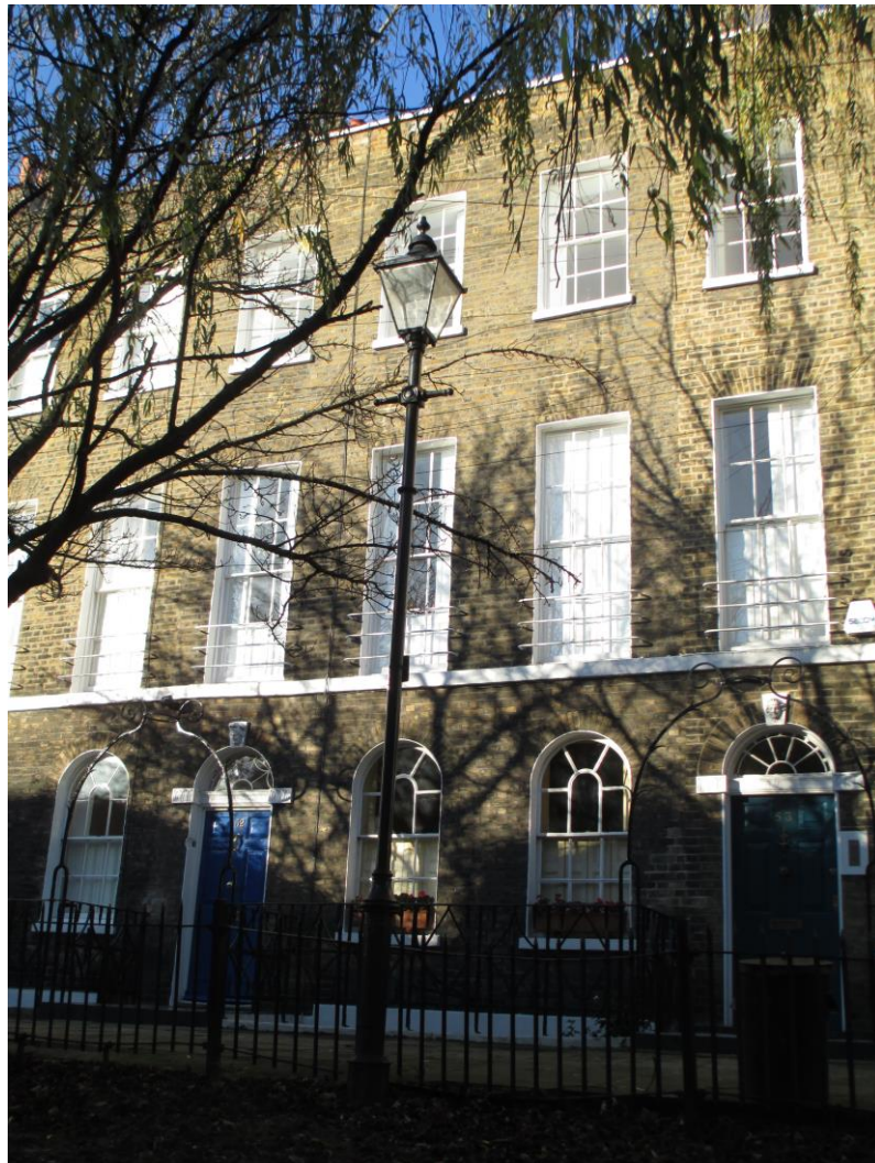
Image 2 - View of front elevation of site
