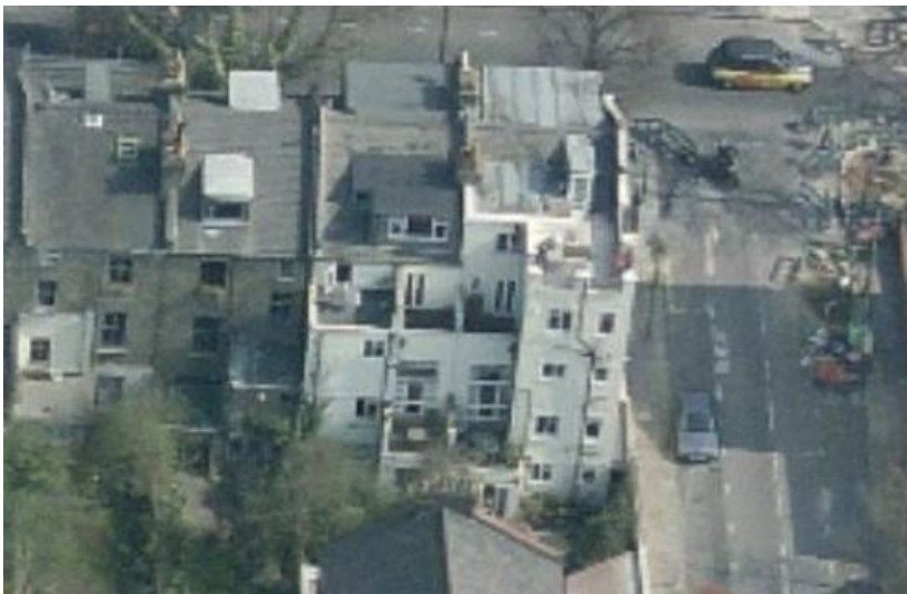
Image 1: Aerial photograph showing the rear elevation
